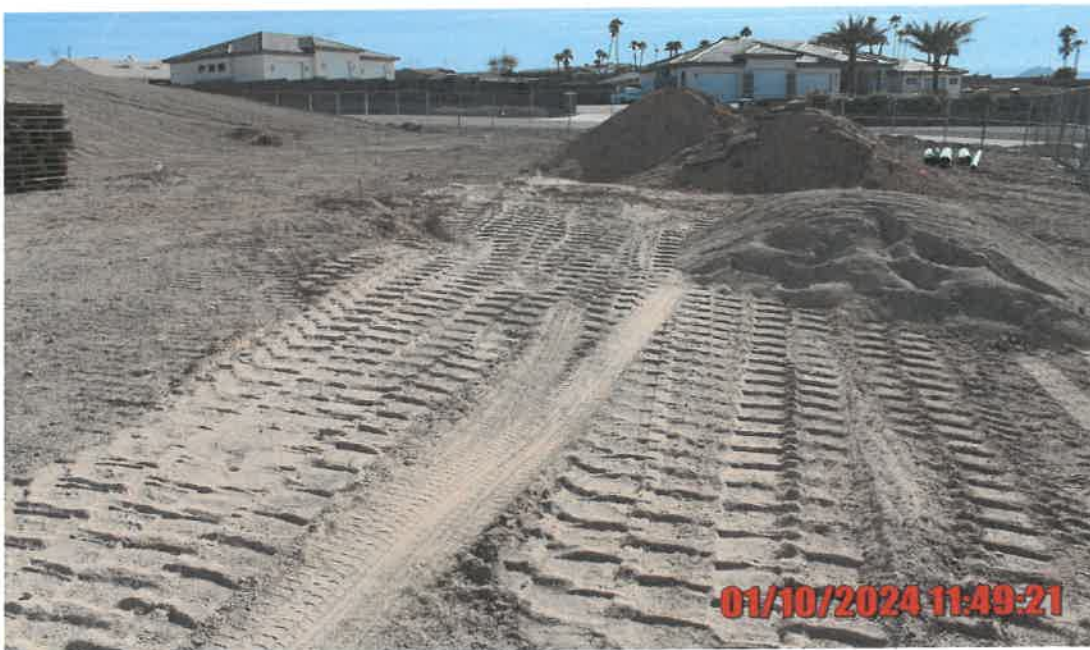
Photograph # 2 Alleged Violation # 1, 2 View looking south at dry, loose and powdery site soils with no available BACM at a project site without a valid dust control operating permit on lot #006, 724 N Naples Street. Photo taken by Senior AQS, Katrinka Byers.
