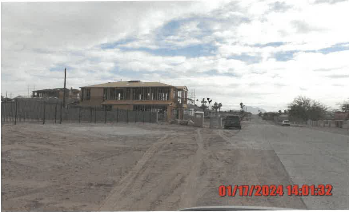
Photograph # 7 Alleged Violation # 1, 2 View looking south at dry, loose and powdery site soils with no available BACM during a follow-up visit. Photo taken by Senior AQS, Katrinka Byers
